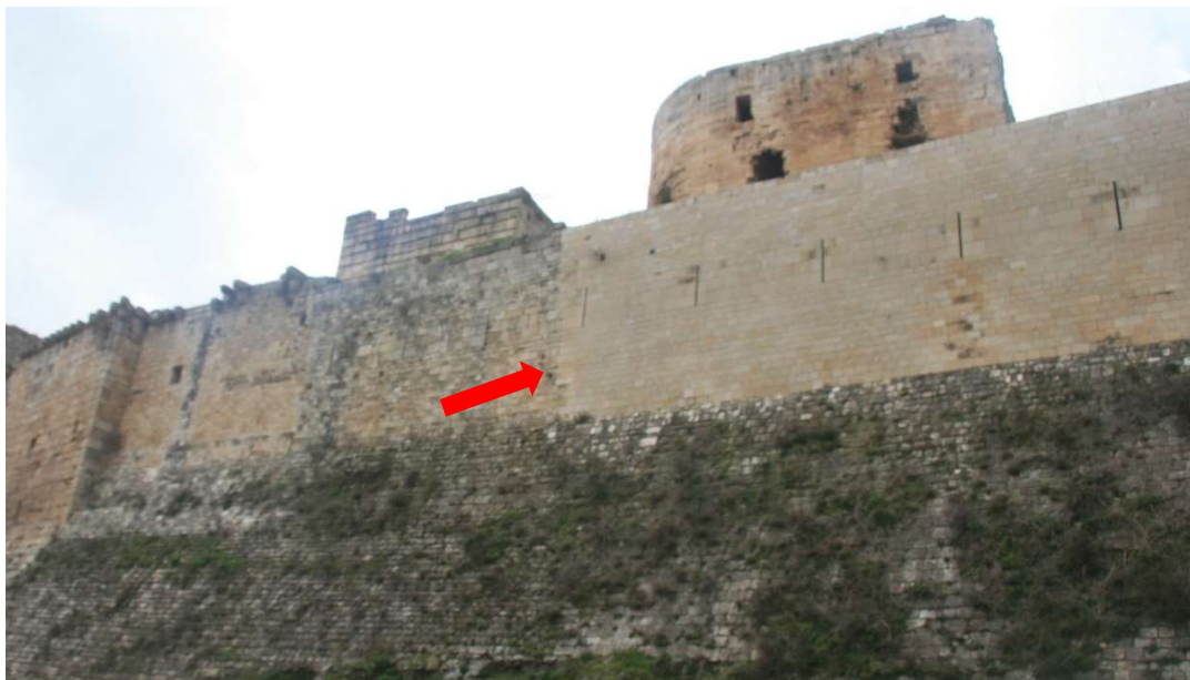
Figure 3. 20 The restoration work of the Building (103) in 2006
