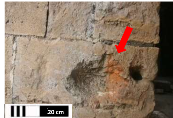
Figure 4. 2. 23 Deposition of orange material on the damaged parts by bullet at Building (19)
