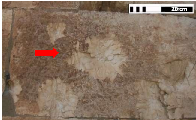
Figure 4. 2. 3 Loss in stone material case in stone exposed to missiles fragmentation
