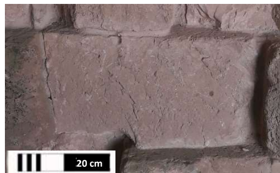
Figure 4. 2. 21 Eroded surface in Building (35)
