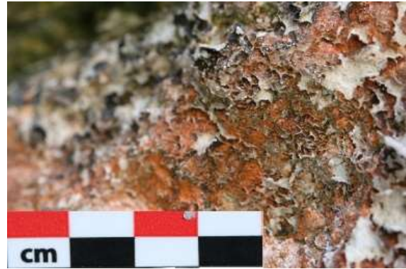
Figure 4. 2. 7 The microorganism colonization on third pillar from west of the first northern row of Pillar of Building (4) (east face)
