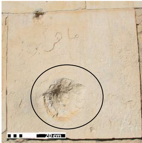
Figure 4. 2. 2 Powdering case in stone
