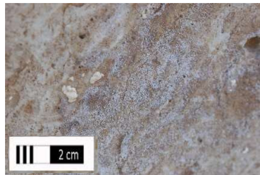
Figure 4. 2. 14 Salt efflorescence on a stone surface located in the first floor. The salt source is from sea spray effect
