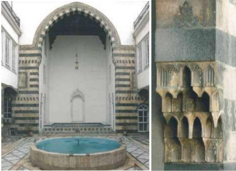
Figure 102 The iwan in al-'Aqqād House and the muqarnas of the iwan arch (Mortensen & Weber 2005: 238-245)
