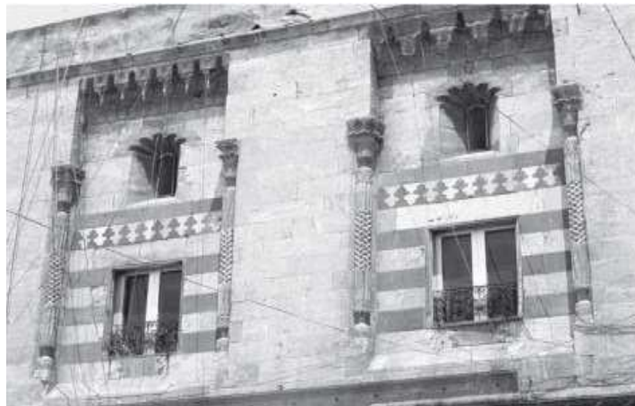
Figure 155 The interior Northern facade of al-Jumruk Khan (Watenpaugh 2004: 303)
