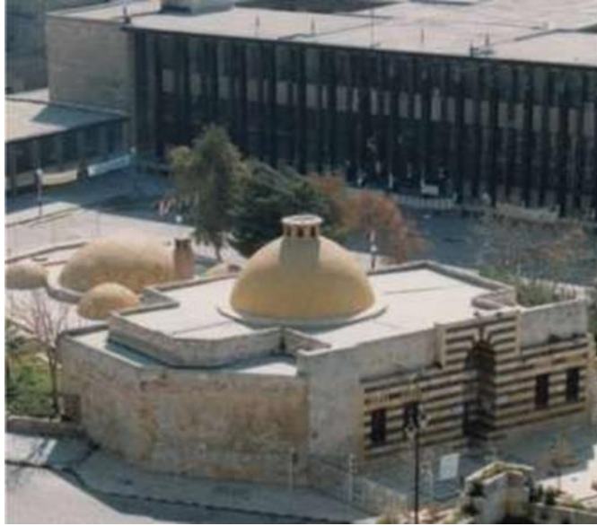
Figure 161 General view of Bahram Pasha Hammam (al Ḥumṣī 1983: 173)
