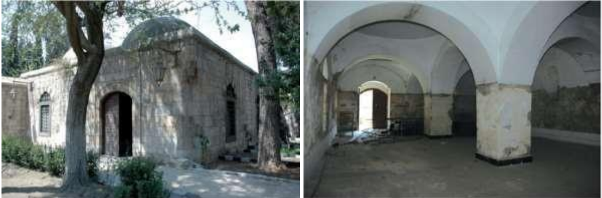
Figure 30 The exterior and interior view of the caravanserai (Güçhan & Kuleli 2018: 14)
