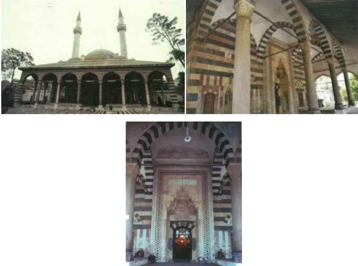
Figure 27 The facade of al- Suleimaniyya Mosque (Kasmo 2017: 210-212)
