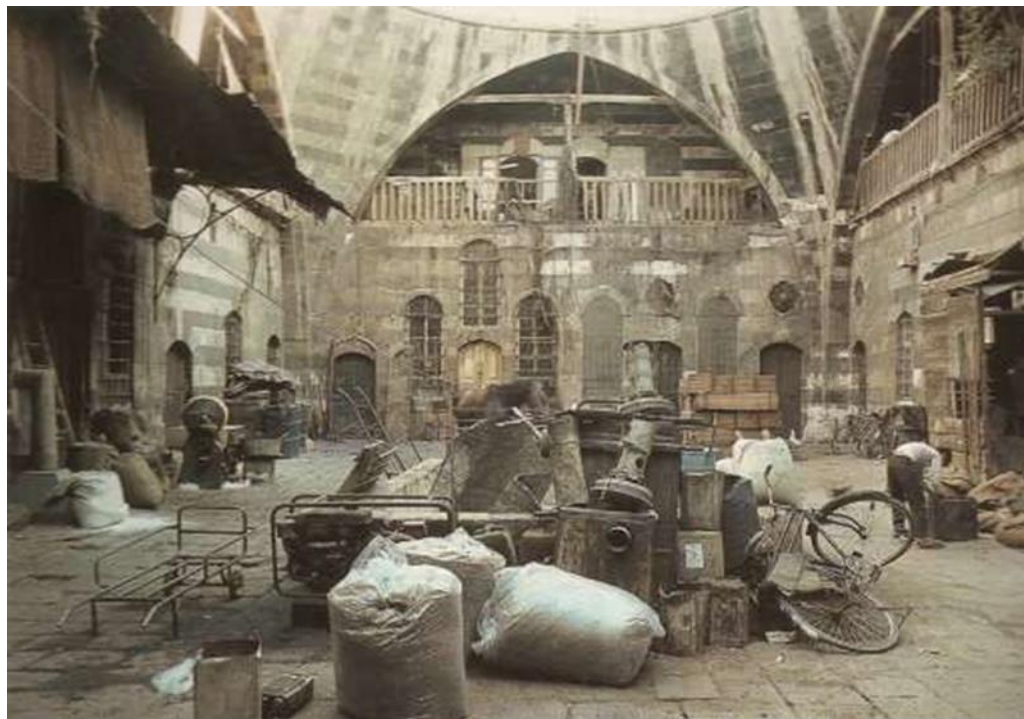
Figure 84 The courtyard of Khan Suleiman Pasha al-'Azim Khan and the pendentives which held the domes (Degeorge 2005: 195)
