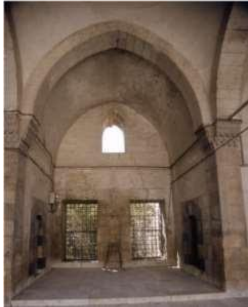
Figure 146 The eastern iwan in al-Bahramiyya Mosque (Kasmo 2022: 28)
