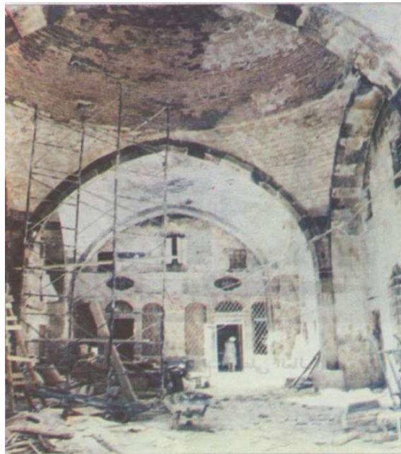
Figure 79 The domed courtyard of al-Tutun khan during the reconstruction (al-Shihābī 1990:216)
