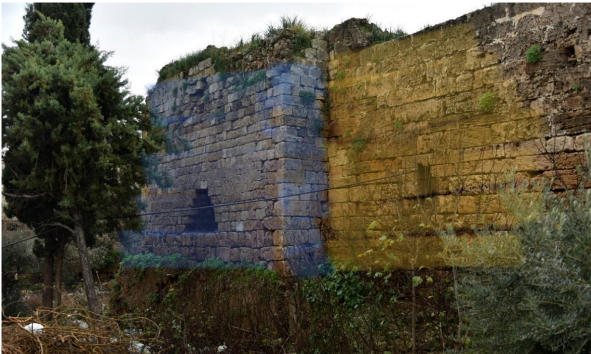
Fig. 45-Junction between wall 15 and the tower 16 on the eastern façade of the castle enceinte.
