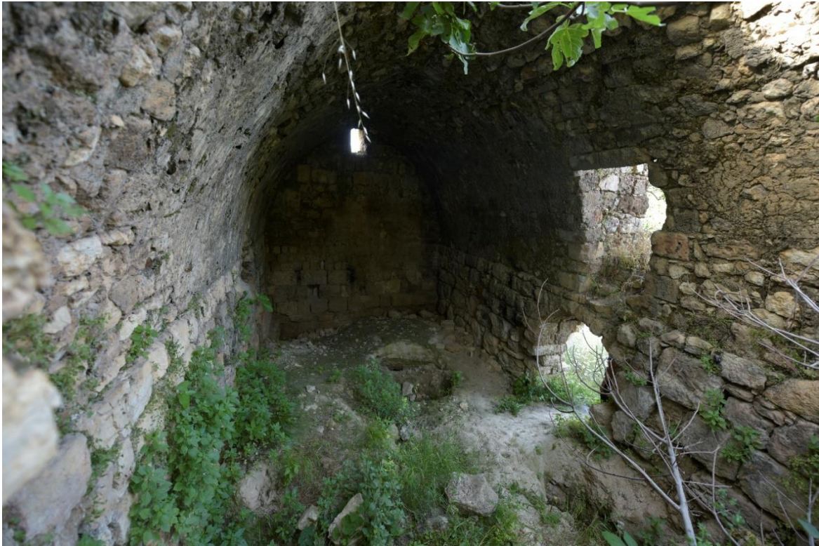
Fig. 121-Inner space showing the western inner wall.
