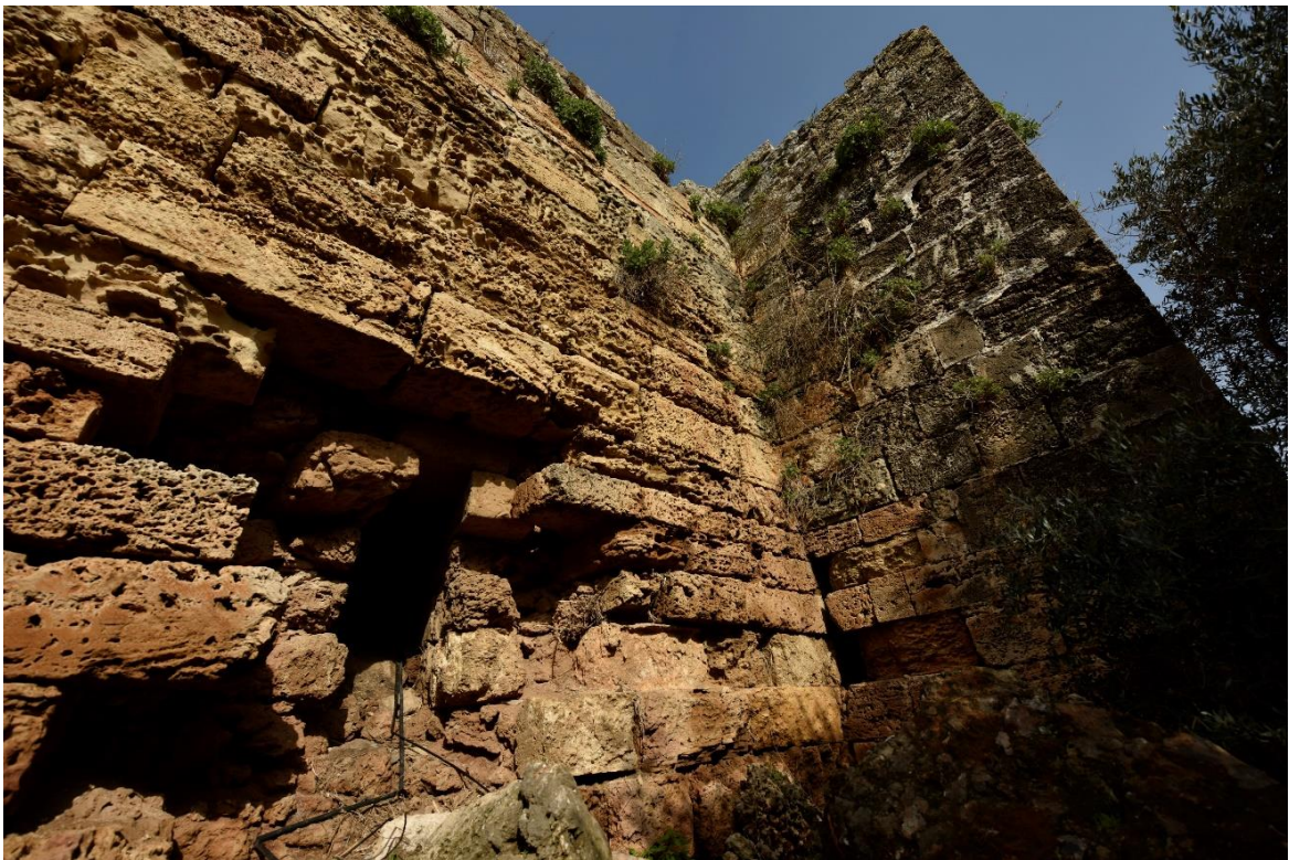
Fig. 18-Western façade of tower 4.
