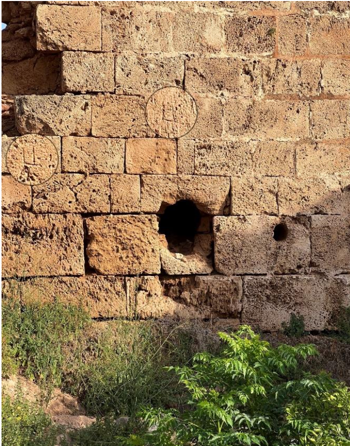
Fig. 37-Bottom corner opening in the north façade and some masons' marks visible.
