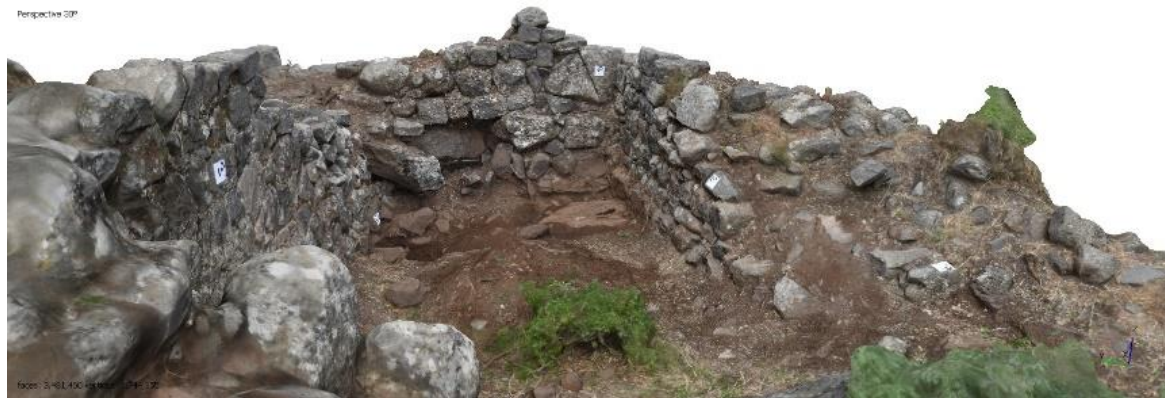
Fig. 133-View of the western wall of the main tower B4.
