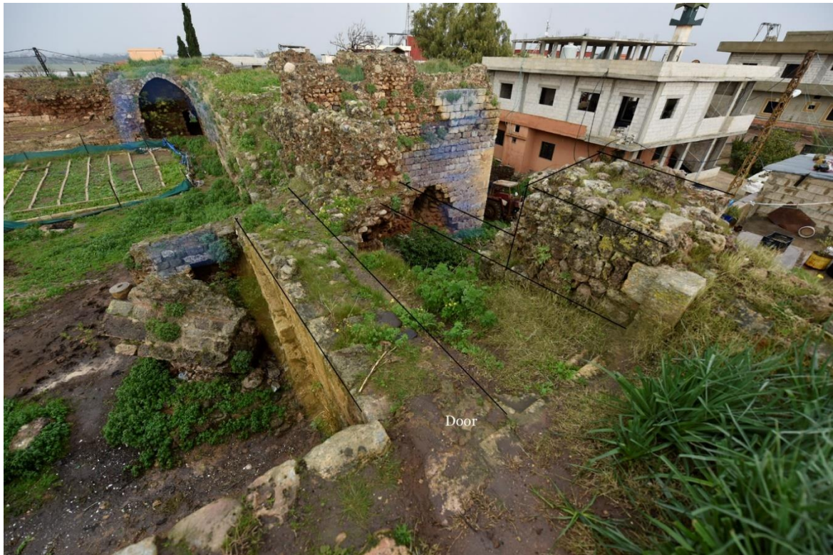
Fig. 57-Overview of the eastern wall of the castle.
