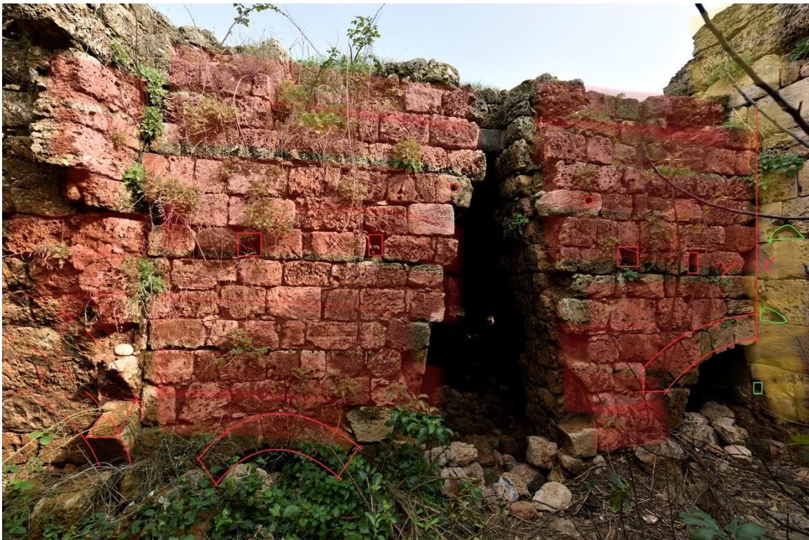
Fig. 27-Eastern wall of space 8.o.
