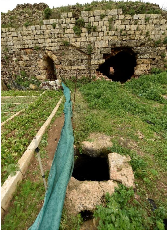
Fig. 14-Cistern opening in the courtyard.
