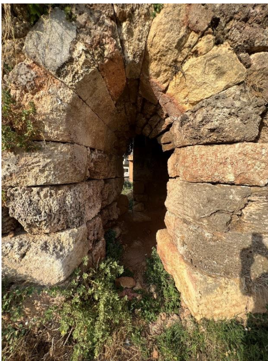
Fig. 55-Blocked arrow slit with the latrine turret in space 19.o.
