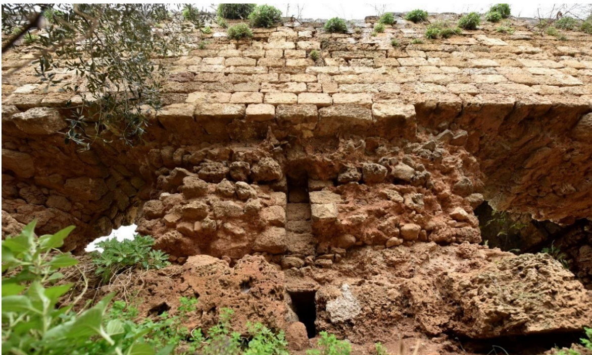
Fig. 53-Eastern face of wall 18 showing a shaft.
