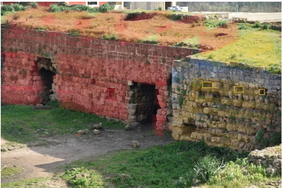
Fig. 13-Northern façade, of space 3.0 and 5.0.
