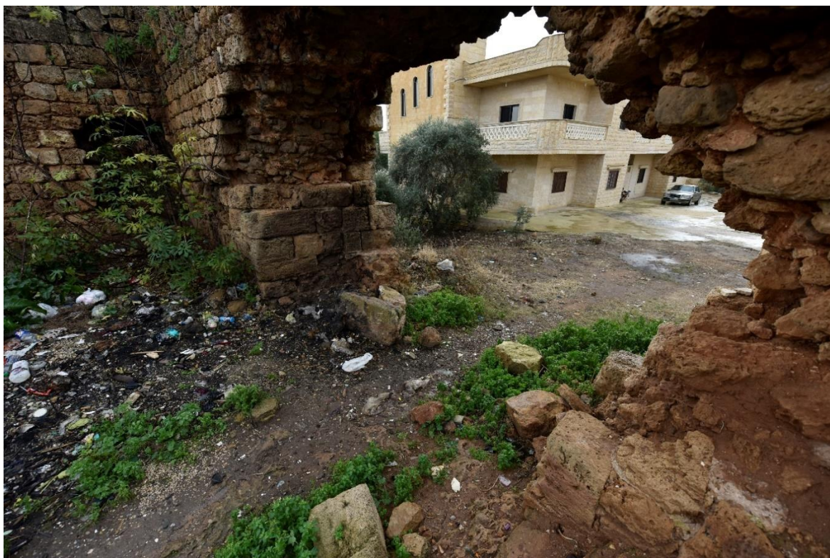
Fig. 4-Contemporary opening in the western wall.
