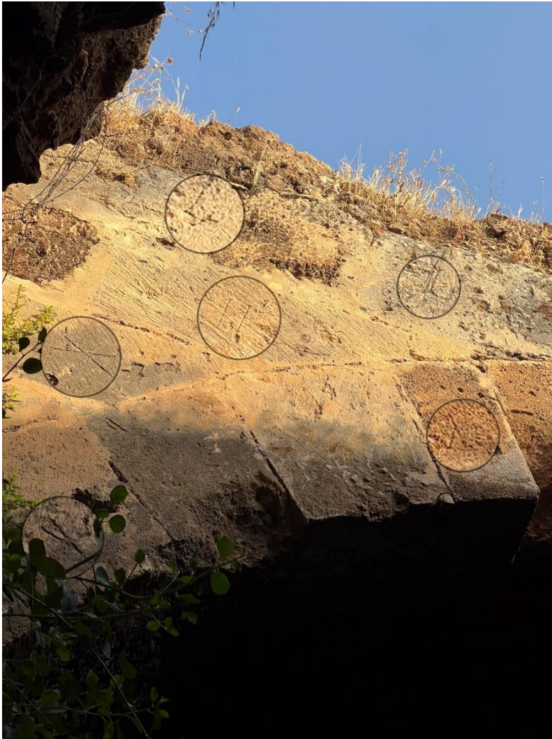
Fig. 62-Northern face of tower 4 showing Medieval assembly Marks.
