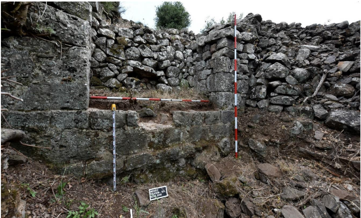
Fig. 94-Gate G3 in the northern wall of the castle. (B. Major).
