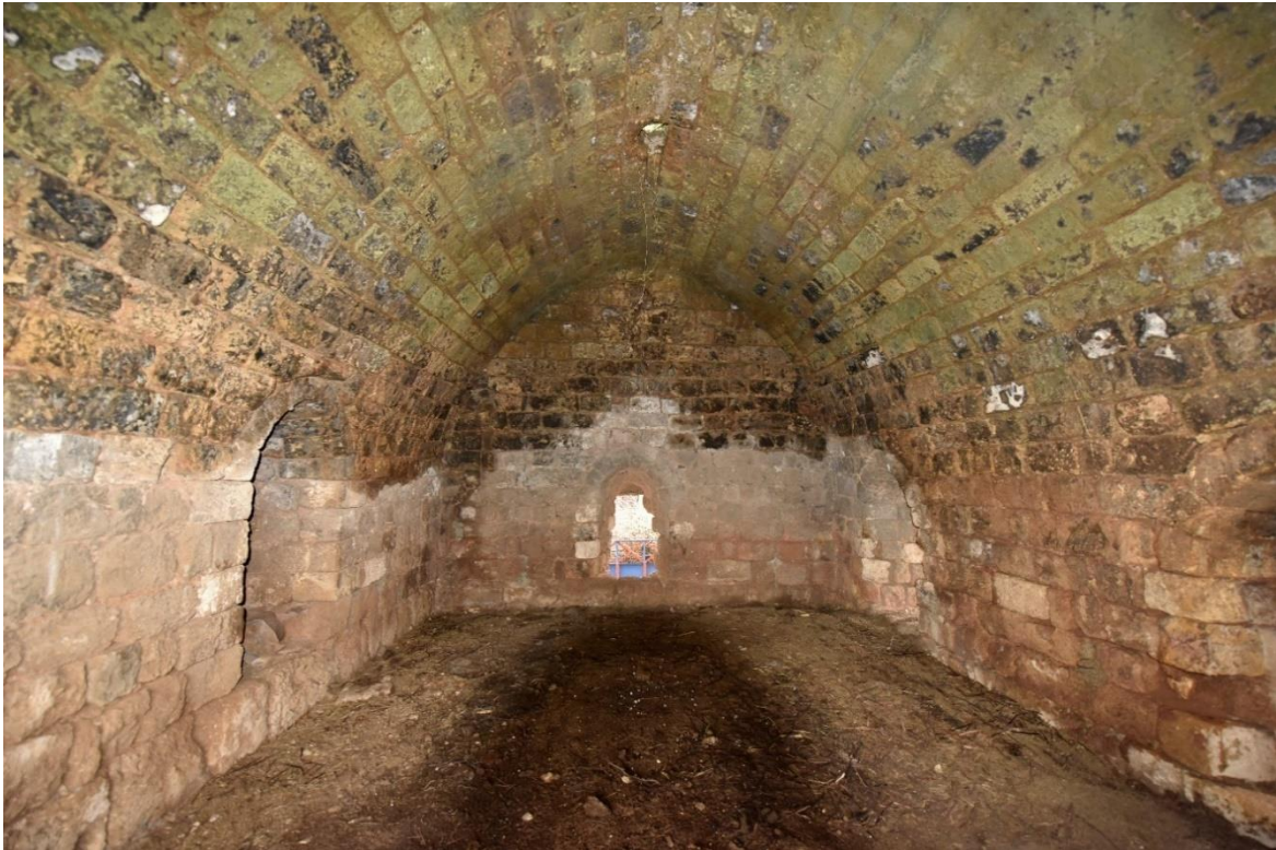
Fig. 50-Inner view of space 19.o.
