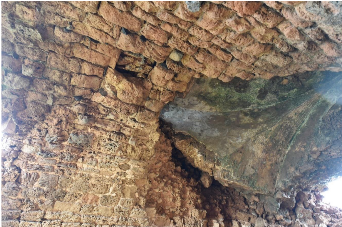
Fig. 34-Inner view of space 12.0.
