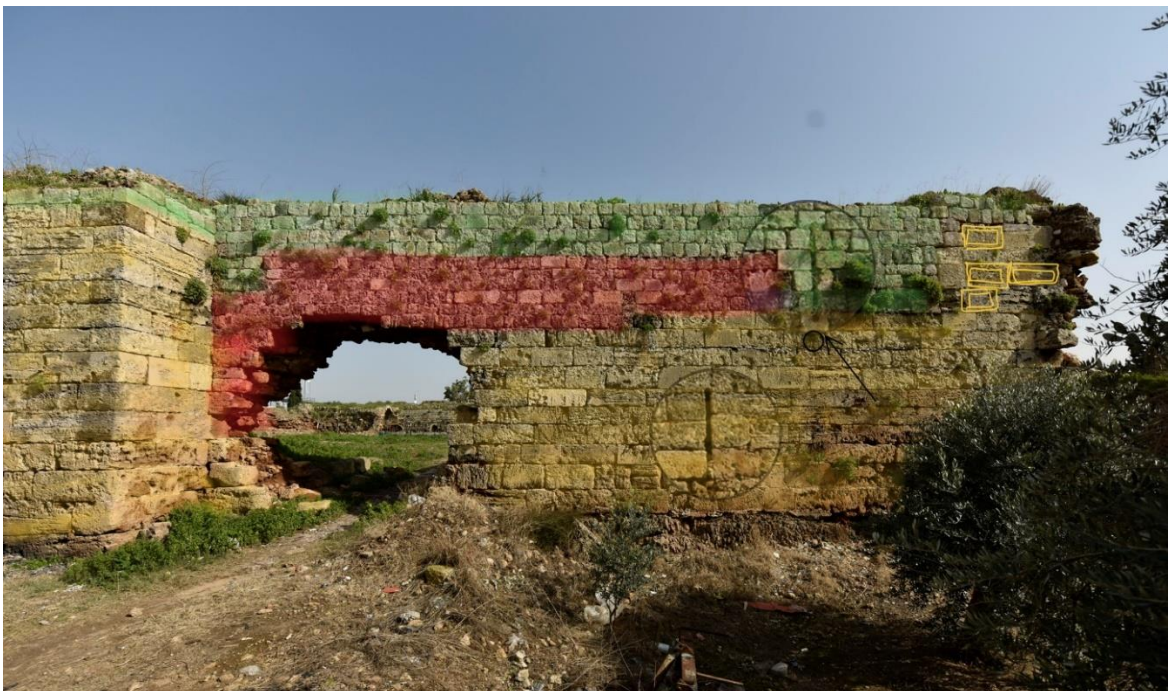
Fig. 9 - Southern section of the western façade.
