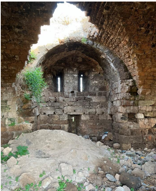
Fig. 22-Inner view of tower 4.
