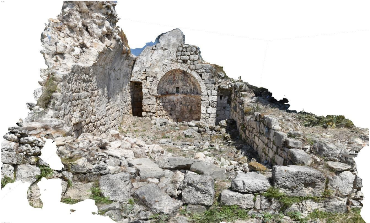
Fig. 152-View of the ruins remaining of the single nave chapel.
