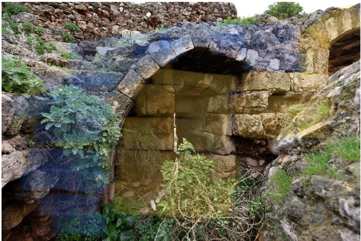
Fig. 42-Guardian space next to the main entrance, space 20.o.
