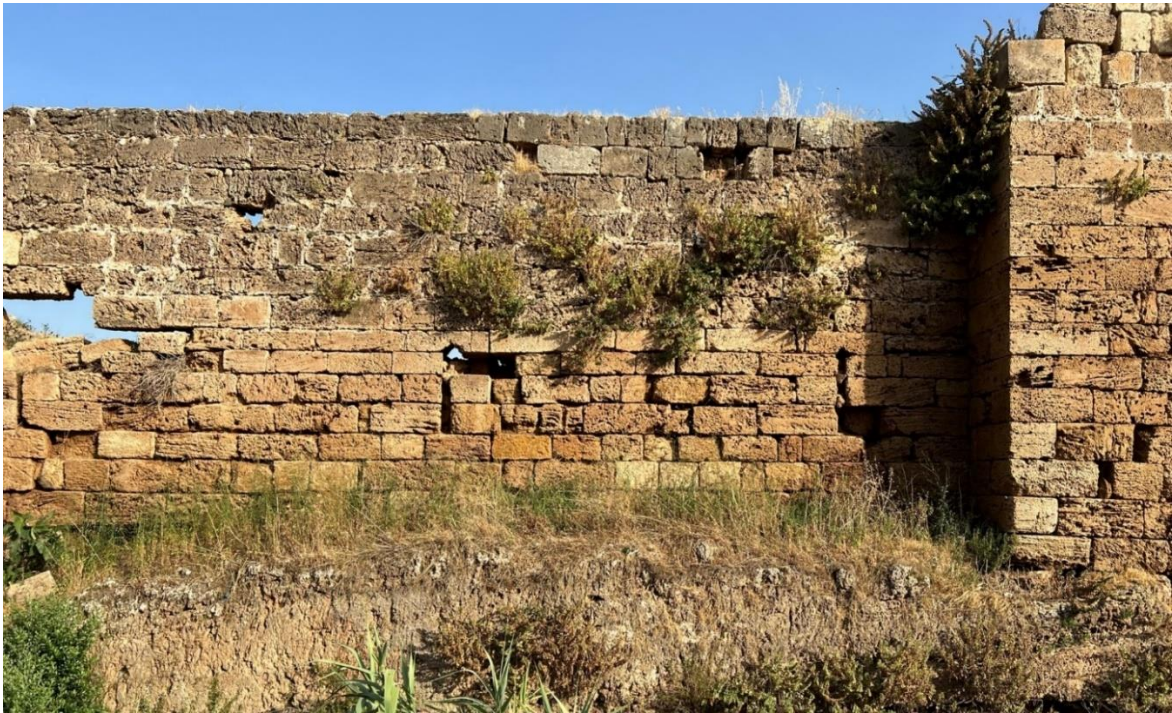
Fig. 38-Northern façade of the wall 15.0.
