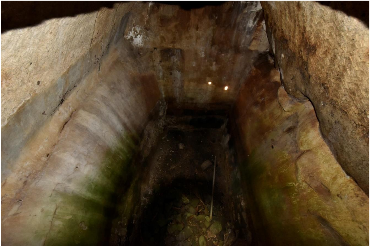
Fig. 93-Interior of cistern no. 2 in the northern bailey of the castle. (B. Major).
