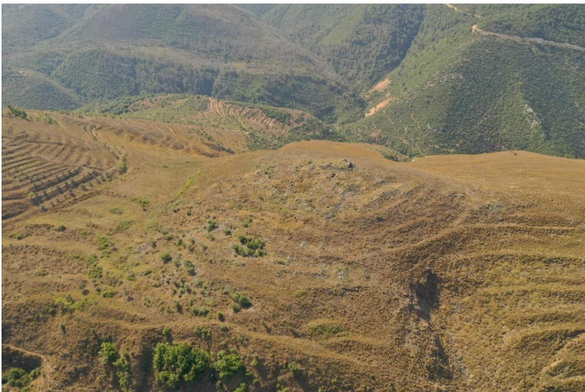
Fig. 102-Aerial photo showing the houses on the hill on a lower level than the tower.
