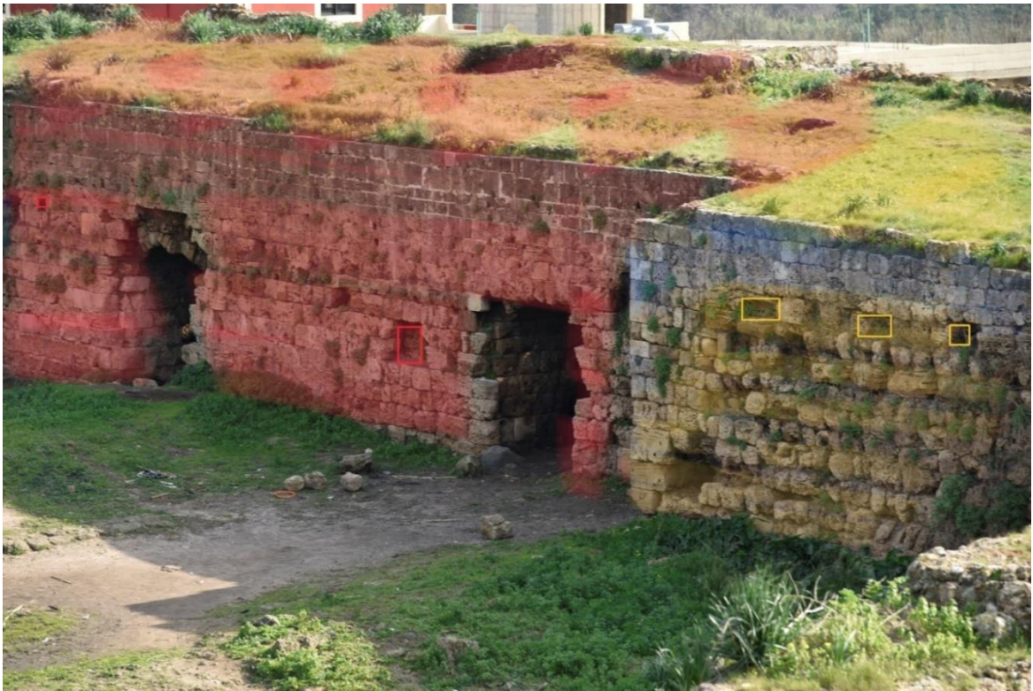
Fig. 44-Northern façade, of space 3.o and 5.o.
