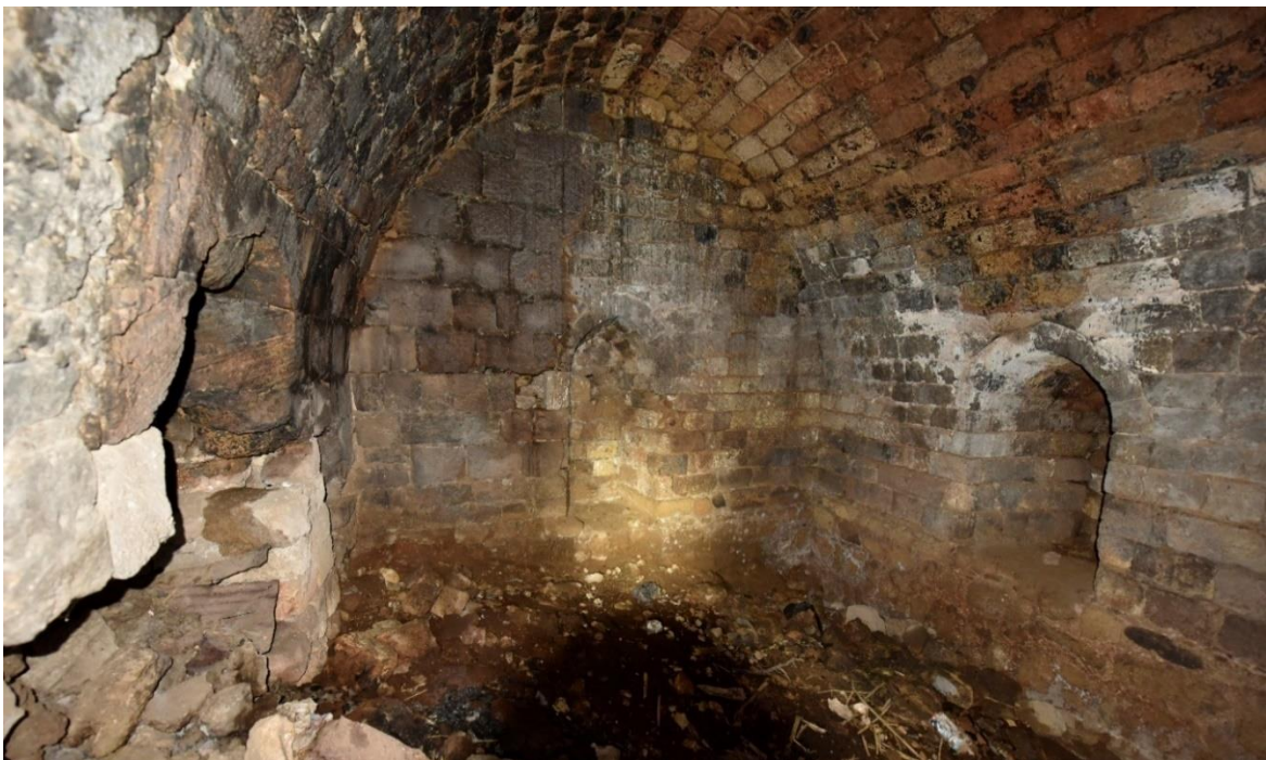
Fig. 7-Tower 2.0 interior looking southeast.
