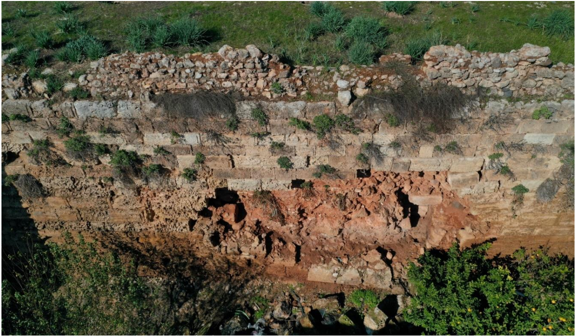
Fig. 15-Aerial photo showing part of the southern façade of the castle with bossed ashlars.
