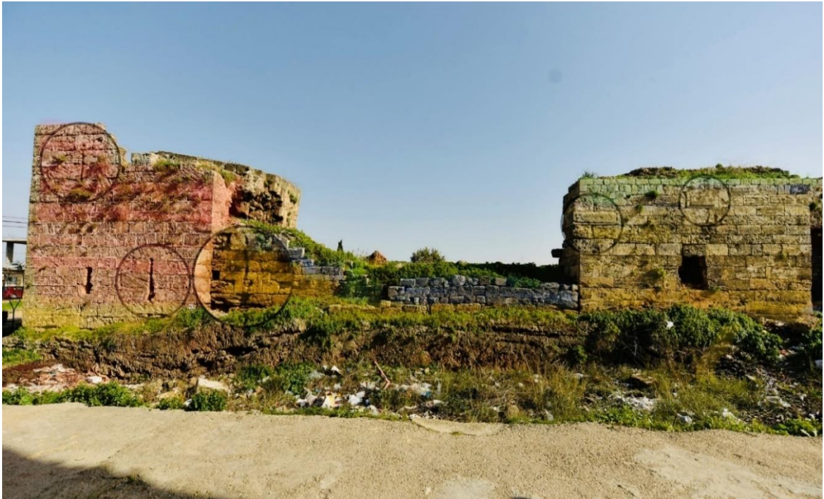
Fig. 8 – Northern section of the western façade of the castle.
