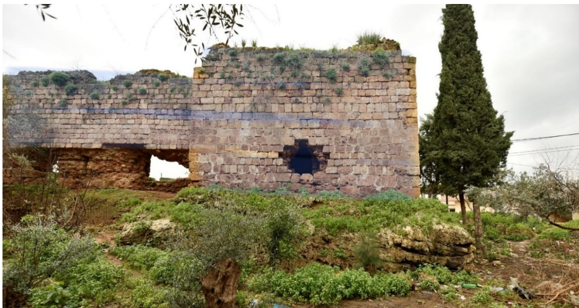
Fig. 46-Eastern façade of tower 16.
