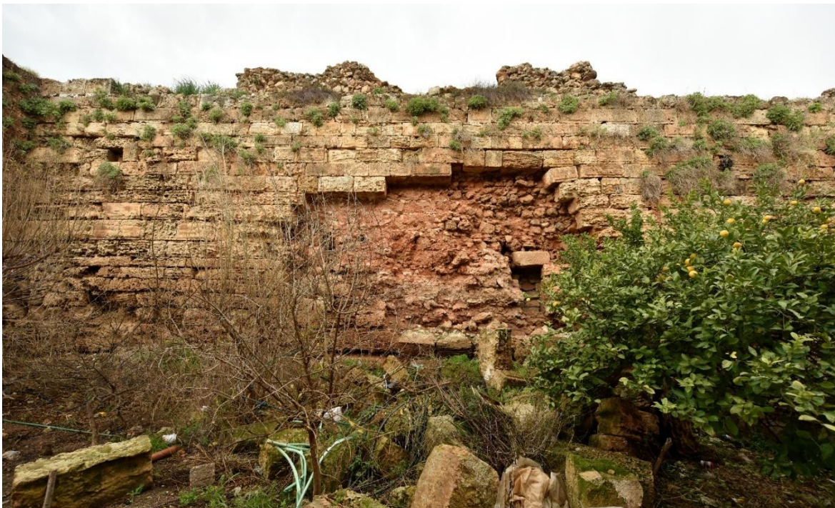
Fig. 16-Southern façade of the castle between towers 2 and 4.
