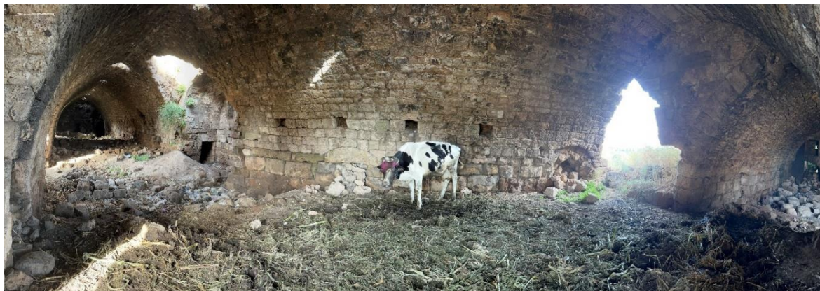
Fig. 24-Current view of space 3.0.
