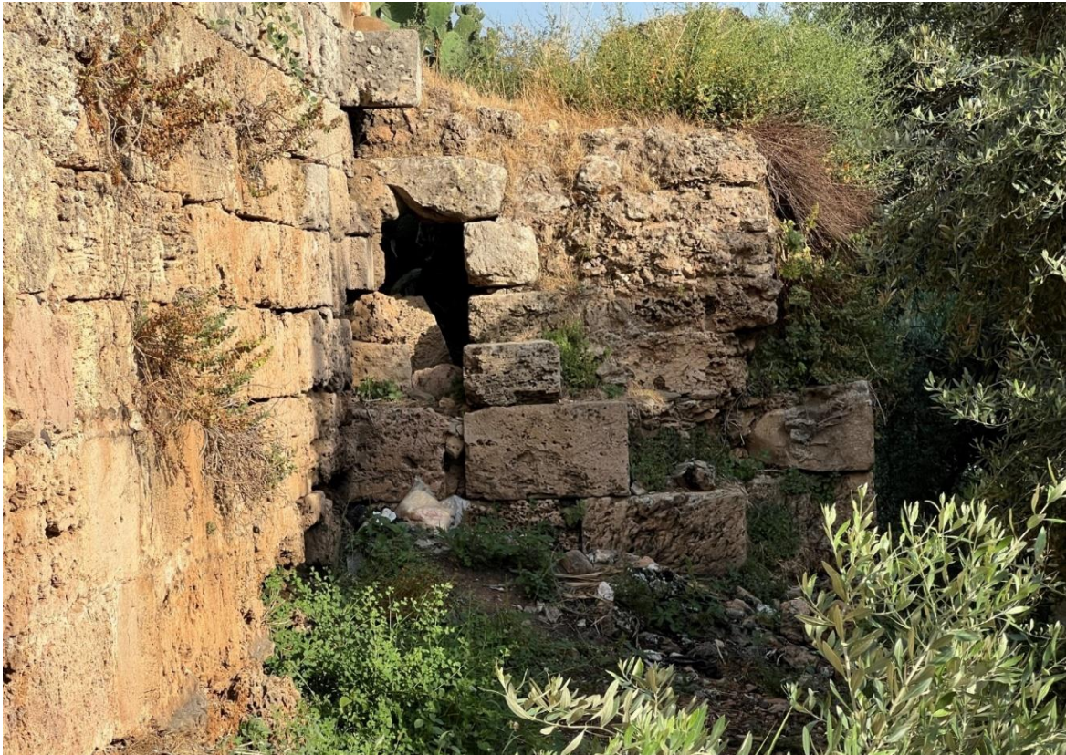
Fig. 5-The remaining northwestern corner of tower 7.
