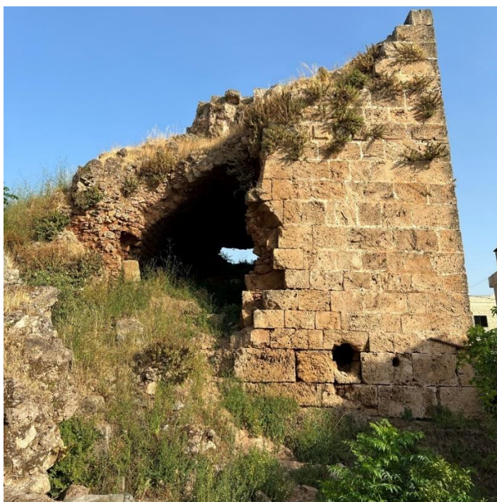
Fig. 36-North face of Tower 12.
