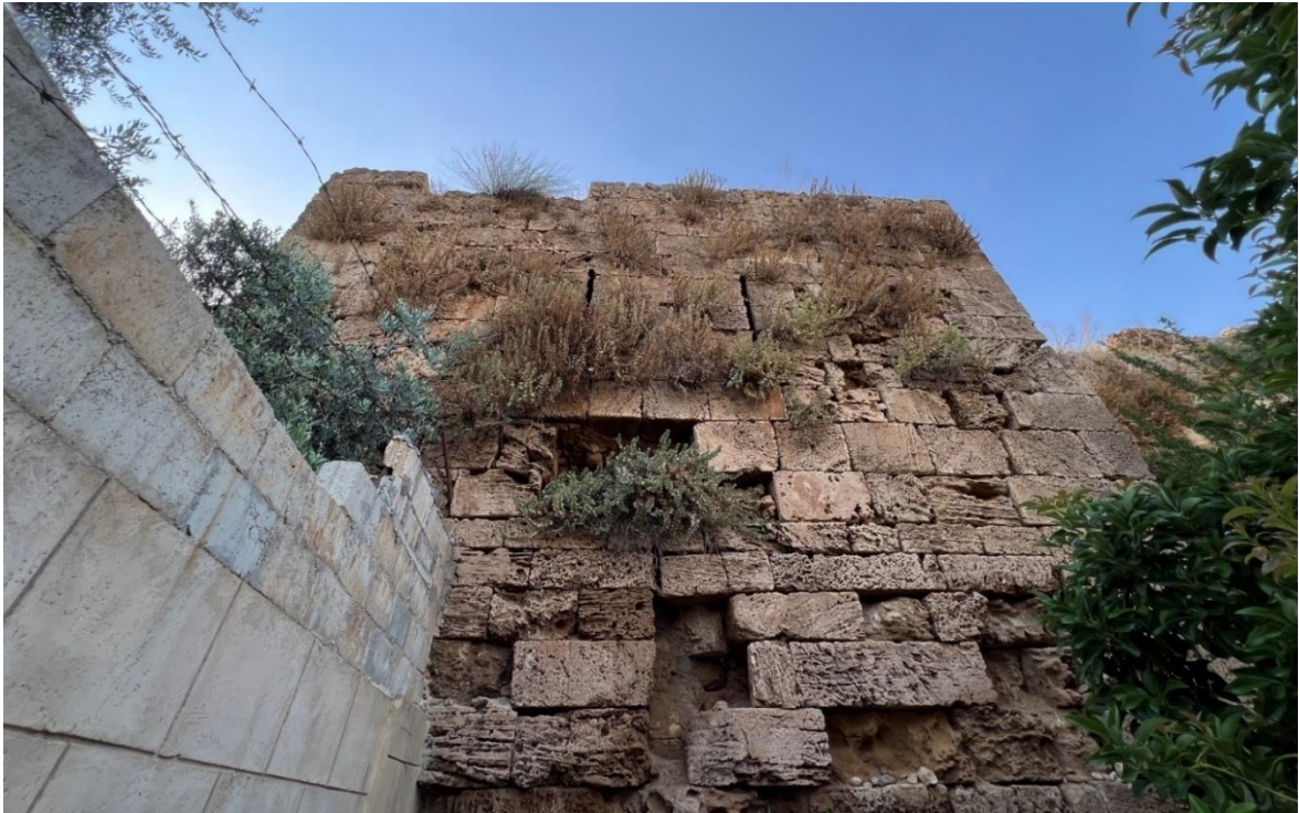
Fig. 17-Southern façade of the tower 4.
