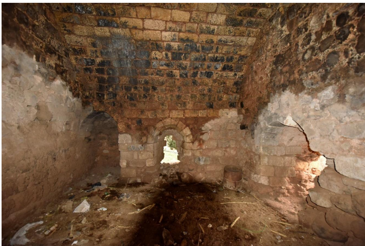
Fig. 47-Inner view of space 16.o.
