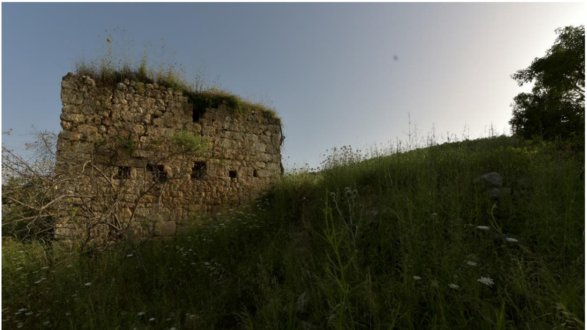
Fig. 119-Western facade of the courtyard house.
