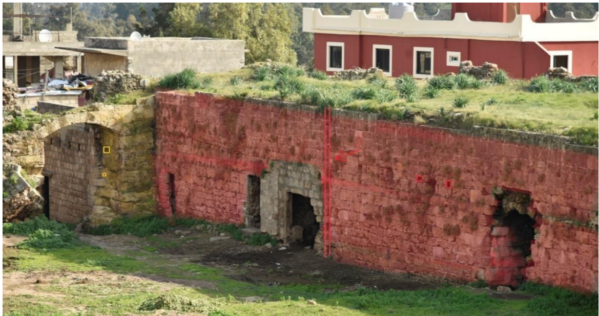
Fig. 43-Northern façade of space 3.o.
