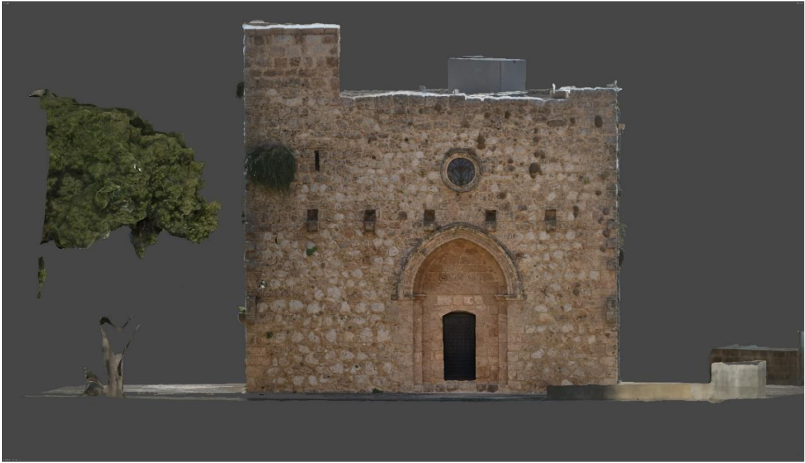
Fig. 148-western facade of the chapel.
