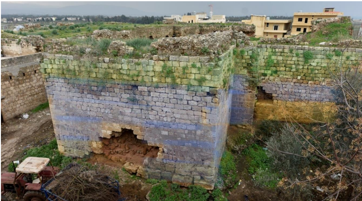
Fig. 52-Eastern façade of Tower 19.
