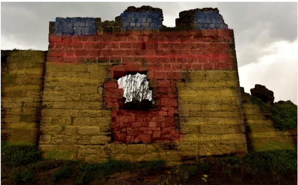
Fig. 39-Northern façade of tower 14.
