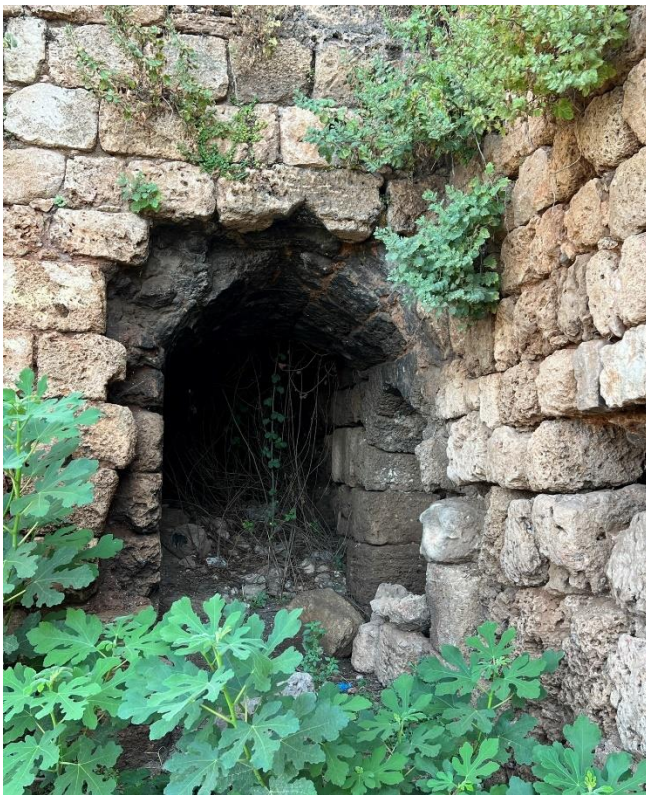
Fig. 29-Door leading to the space 8.o from the courtyard.
