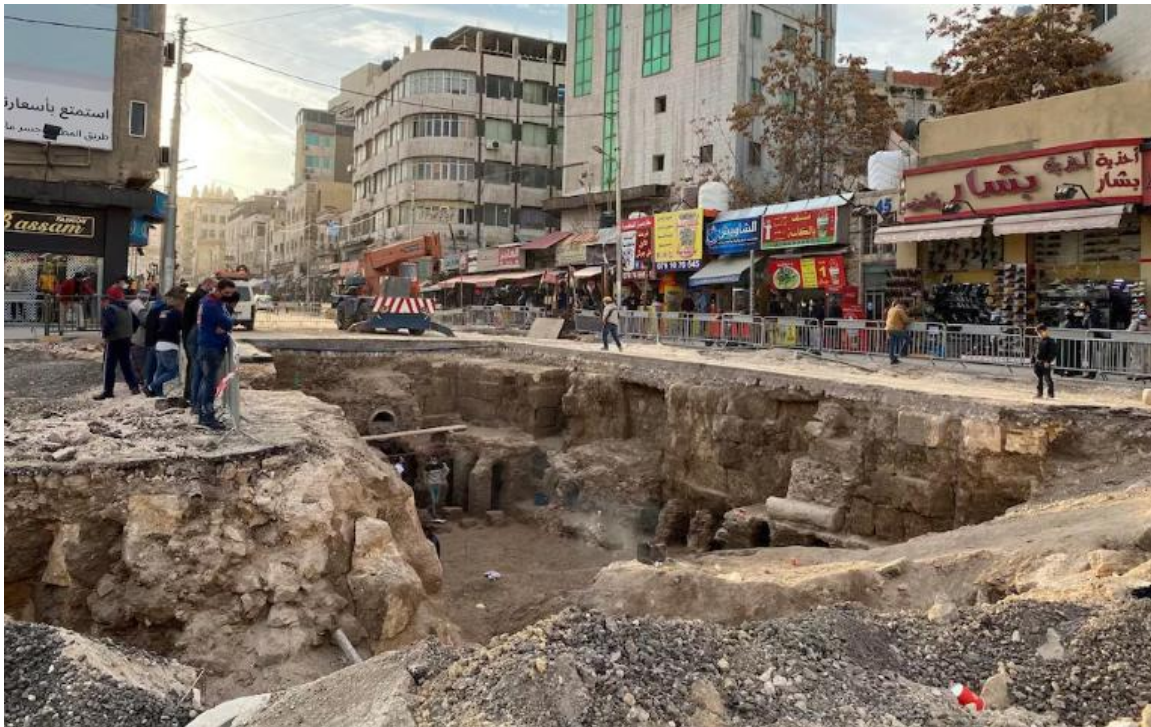
plate 24: Construction work at the so-called Roman bath were uncovered in 2020 an area with shops and local restaurants. Amy McConaghy / The National (Accessed Aug 2023)
